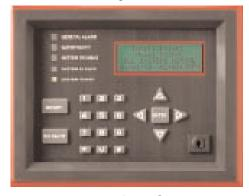
or remote annunciator. System operation can be initiated with a mechanical firefighter's key or a valid 4- to 7-digit operator's code.
